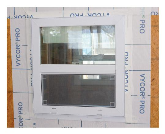
Proprietary adhesive seals and protects details against moisture and air intrusion
