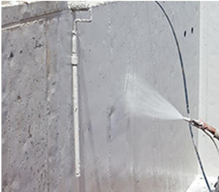
While bustling McCarran International has more than 1,300 slot machines located throughout its existing terminal buildings, the Department of Aviation wasn't gambling with the Terminal 3 airport construction. Because the train station and utilidor tunnel were in the water table, waterproofing was critical. The materials specified provided trouble-free resistance to hydrostatic pressure from the groundwater—and had to be installed during cold and severely hot weather.
